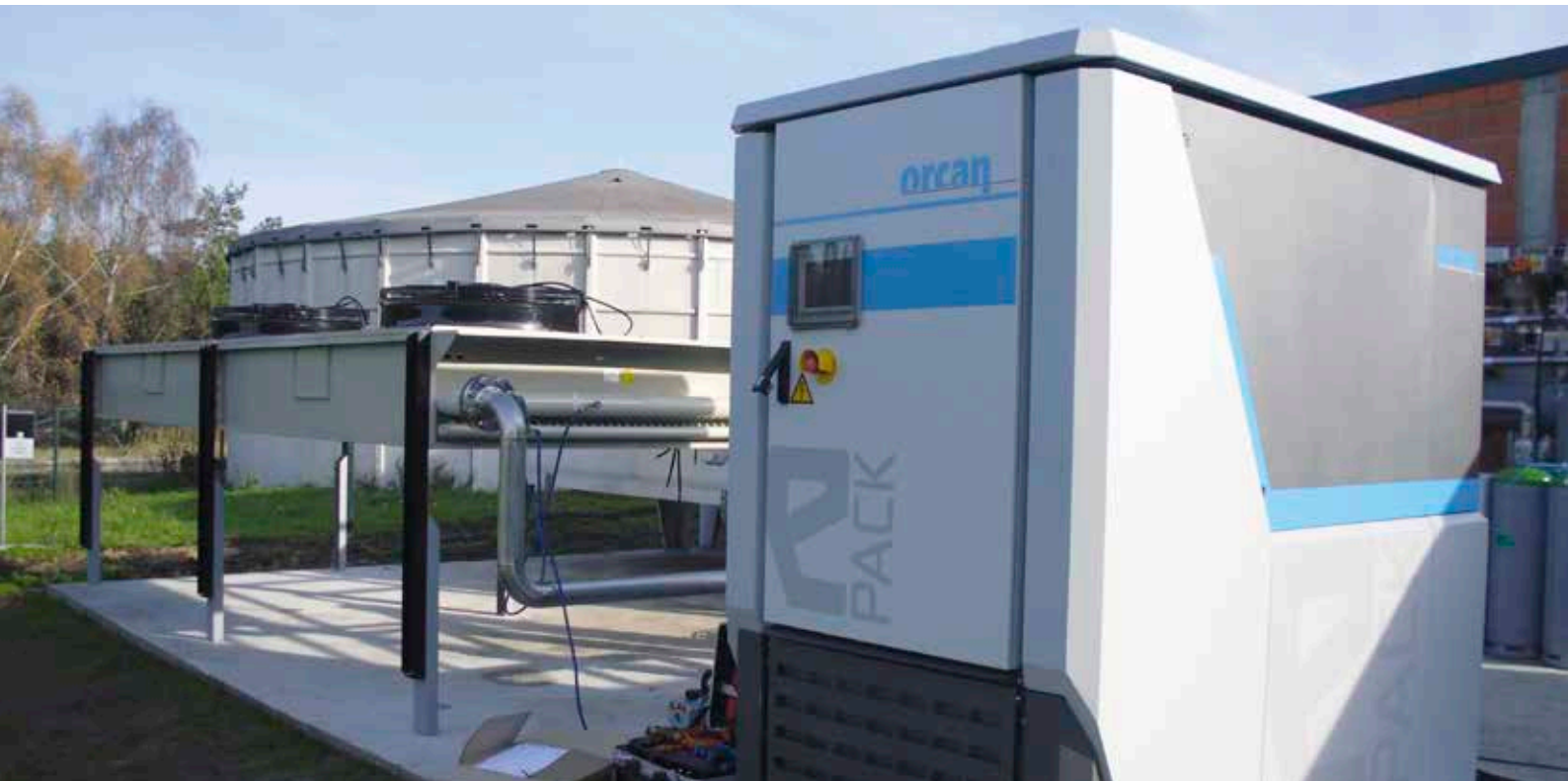
The ePack micro power plant generates power at a rated output of 20 kW from waste gases and the energy contained in engine coolant.
